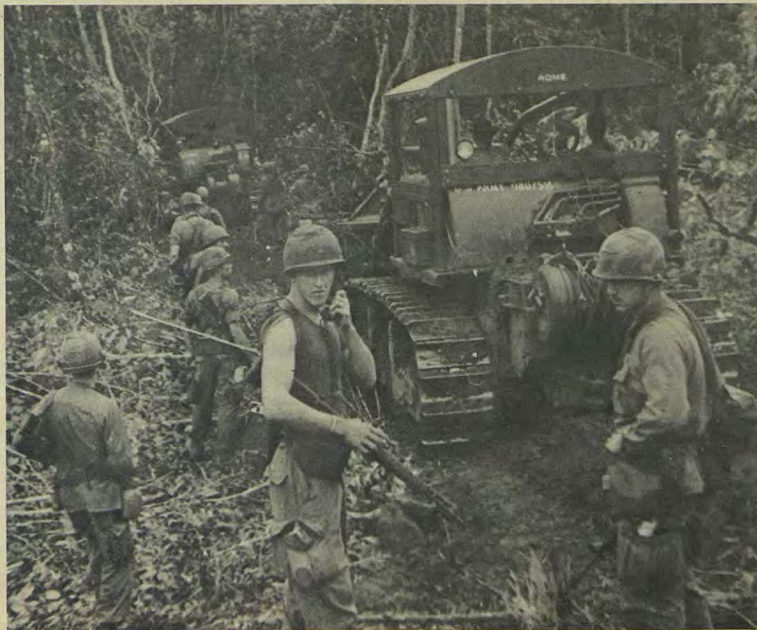
EVE OF DESTRUCTION —Enemy bunkers located west of Landing Zone (LZ) Nicole are about to be destroyed as the heavy equipment crew of HHC, 4th Engineer Battalion, moves into the area on a mission to rid the enemy of fighting positions.
