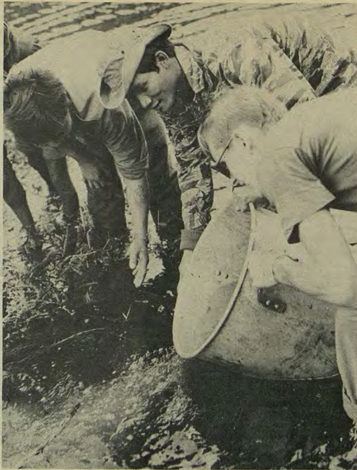
FINISHING TOUCHES —Members of the Fourth Division's G-5 section and the civil affairs team of the 5th Battalion, 16th Artillery help the villagers of Plei Klan Ngol, 25 miles south of Pleiku, to complete their dam construction project. Fish, obtained by the CA teams through the help of the Agricultural Service of Pleiku, are dropped into the artificial lake. The CA teams hope the fish will help to increase the villagers' food consumption. (USA Photo By PFC John D. Warwick)
